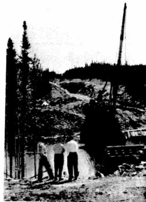
BRIDGE OVER GRASS RIVER: A stiff-leg crane at Mile 13 on the right-of-way of the CNR's H Thompson, scheduled for operation in November cuts on both sides of the site, dumping it into the abutments. Inspecting the project are Inco's chairman, Parker, vice-president and general manager of Canada of the Manitoba division.
